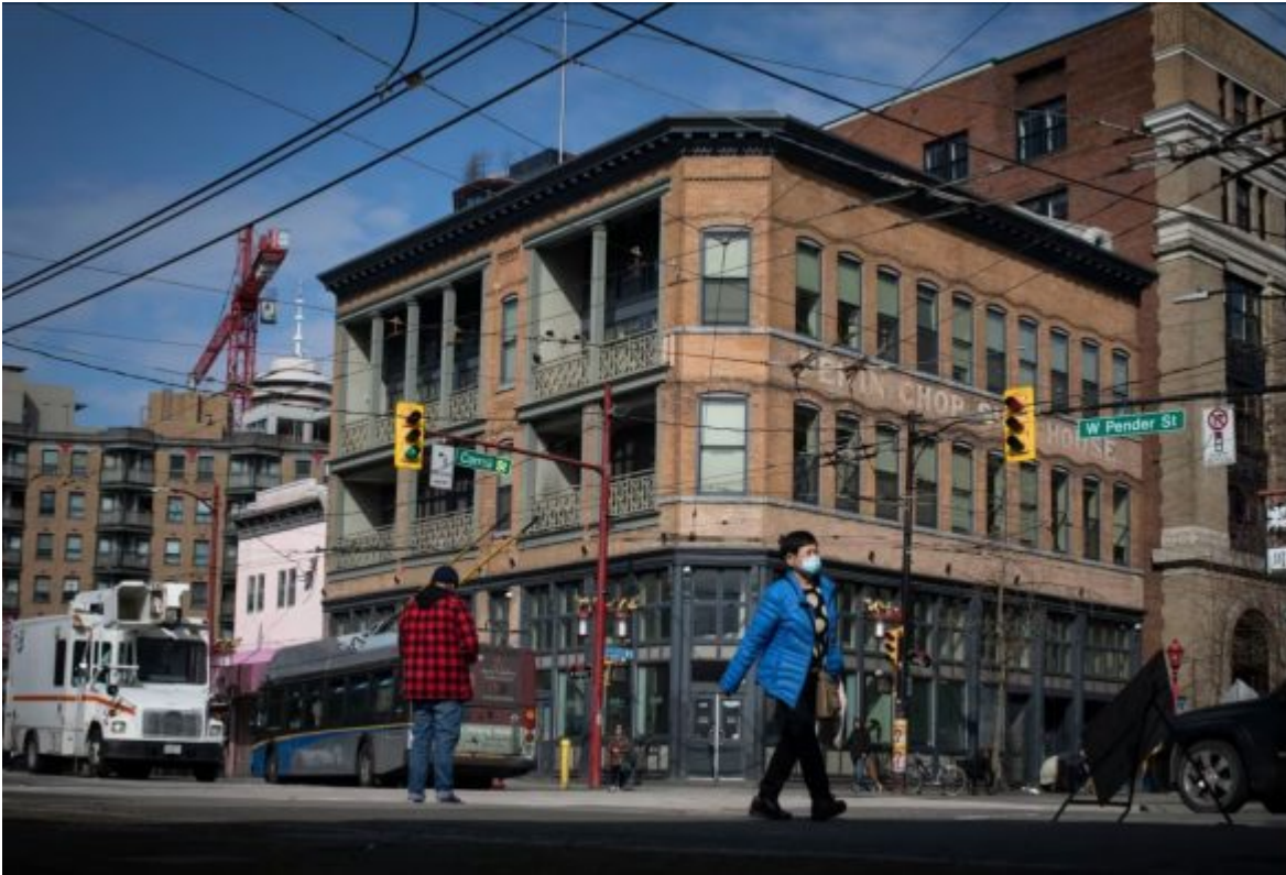
The former Chinese Freemasons building in March 2023. (Ben Nelms/CBC)
